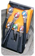
Slide Mechanism Handle UP=|SOLATED
