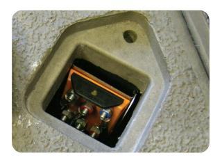
Push down EZ Locate connector mechanism to the lower position. Place enclosure's cover on top and open locate access hatch.
