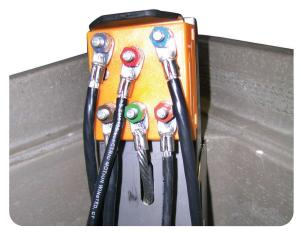
Bonding Harness Or Locate Wires
