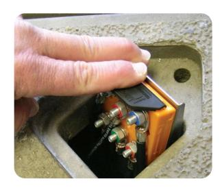
Move test station unit forward and down, securing the EZ Locate test station below the lid of the enclosure.
